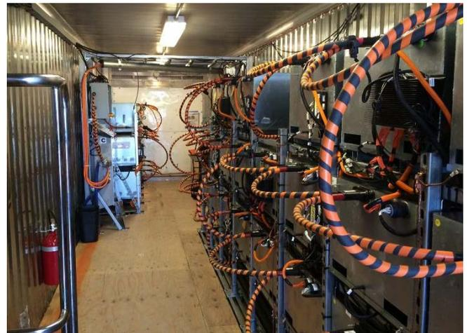
1 MW prototype Grid-Saver™ energy storage system.
